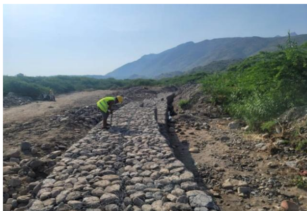
Gabion work in Bajil – Hodeida.
