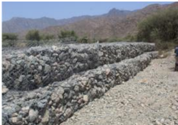
A constructed gabion wall in Lawdar, Abyan
