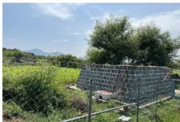
Water Tank Construction in Al-Ma'afer district.
