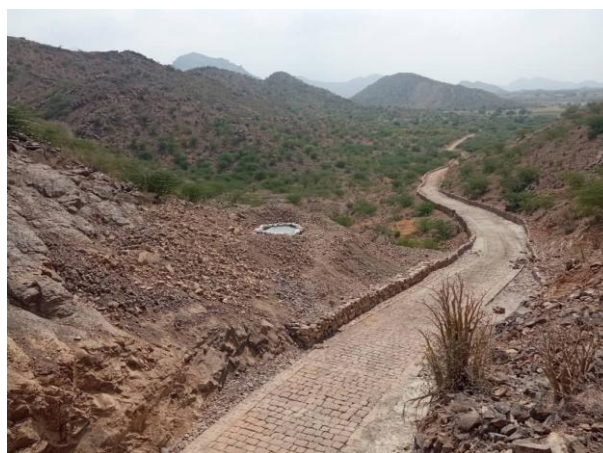
Construction of Road in Al-Qanawis district
