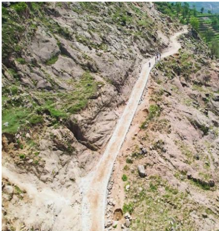
Road pavement in Ash-Shaghdirah, Hajjah Governorate
